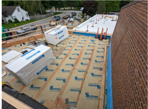
Exterior: View towards the west (roofing in progress)
