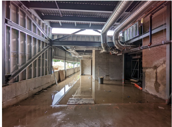
Interior: View towards the west (to the accessible change room)
