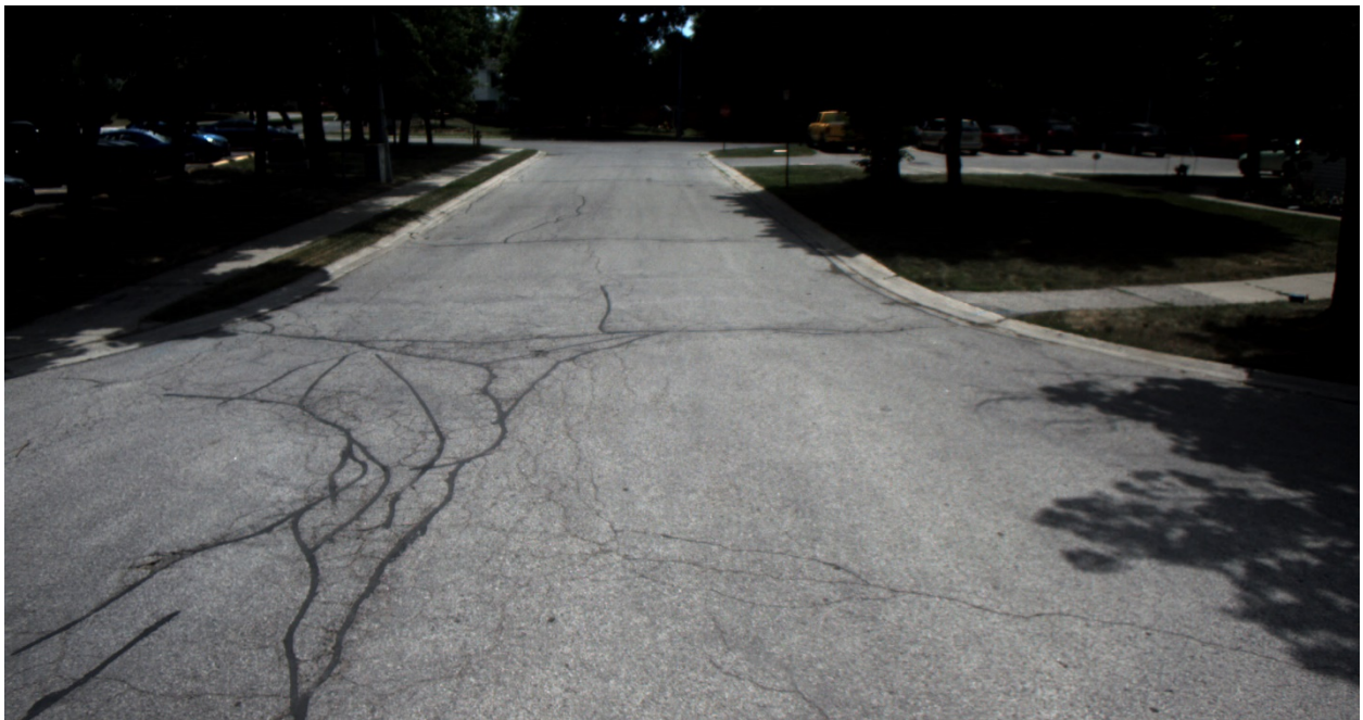
Pavement Condition Poor – PCI 40 – 57
