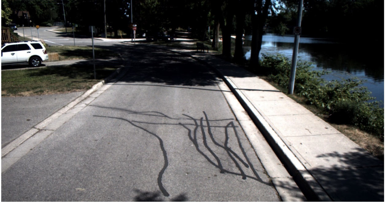
Pavement Condition Poor – PCI 40 – 57
